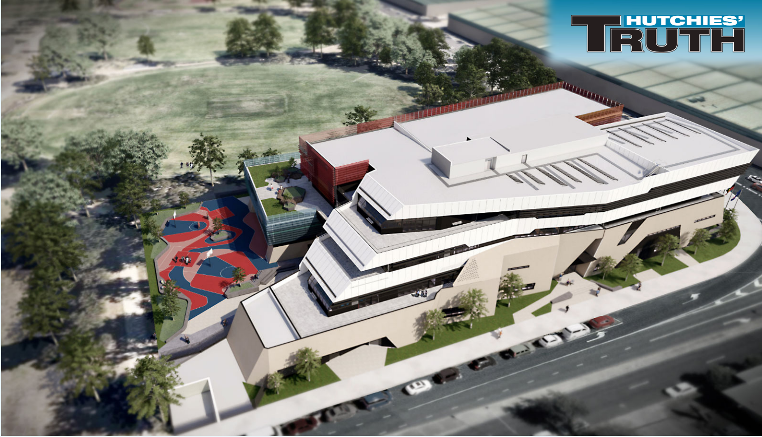
The new Hutchies-built Port Melbourne Secondary College (formerly Fishermans Bend Secondary School) is due to be completed for the start of the 2022 school year.
