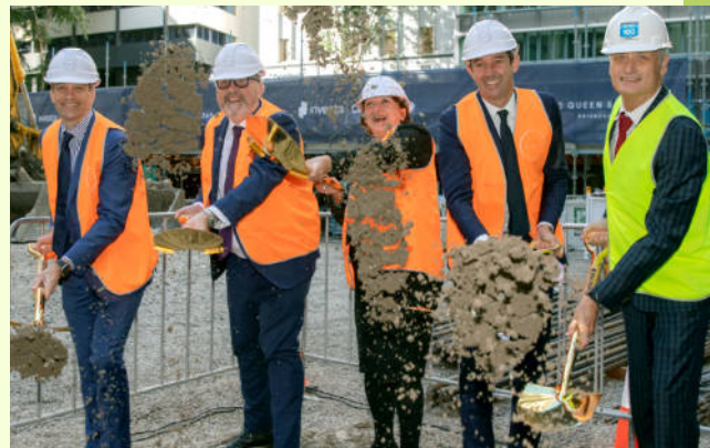
Official party turning the first sod (from left) Bradley Norris and Andrew Borger, representing Charter Hall; Cr Vicki Howard, Brisbane's Central Ward; Brendan Looby, representing Investa; and Scott Hutchinson.
