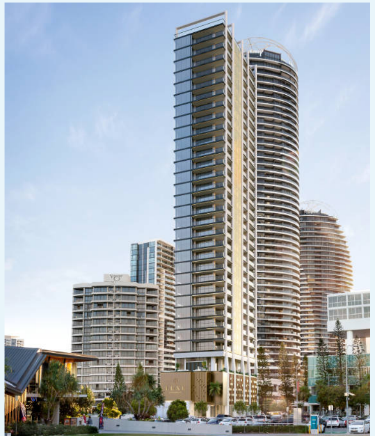
Luxe Broadbeach – a 34-storey beachside residential tower with 28 full-floor apartments.
