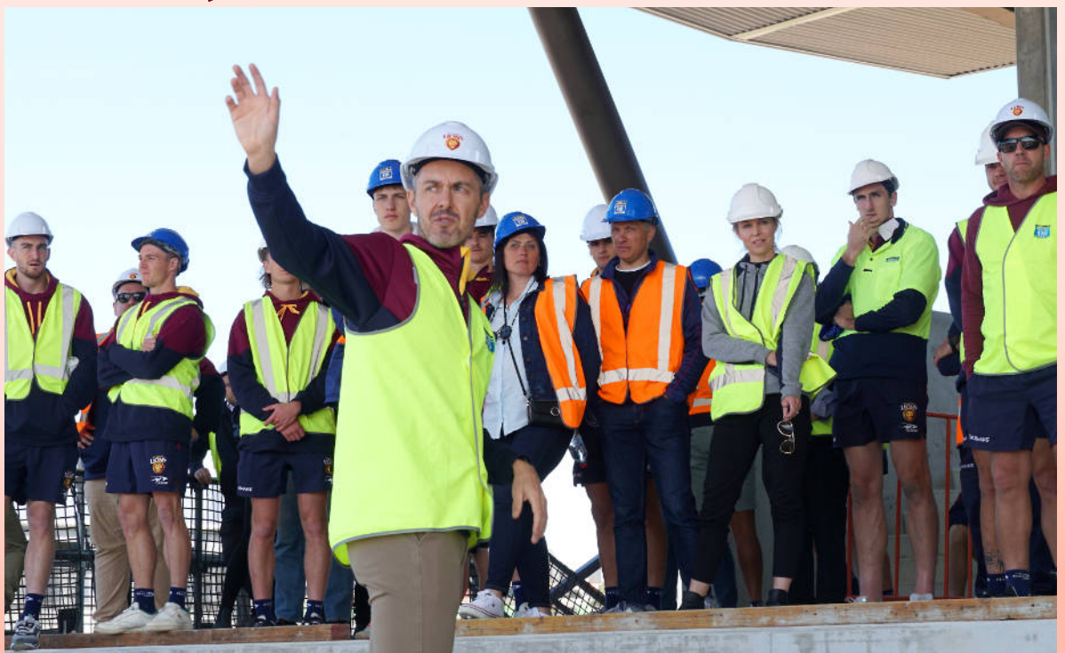
Brisbane Lions and Hutchies inspect progress on the Brighton Homes Arena.
