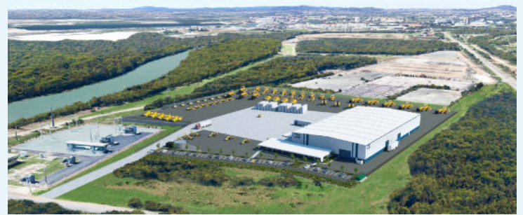
Artist's impression of the new Wallenius Wilhelmsen warehouse and offices under construction by Hutchies for the Brisbane Airport Corporation.
