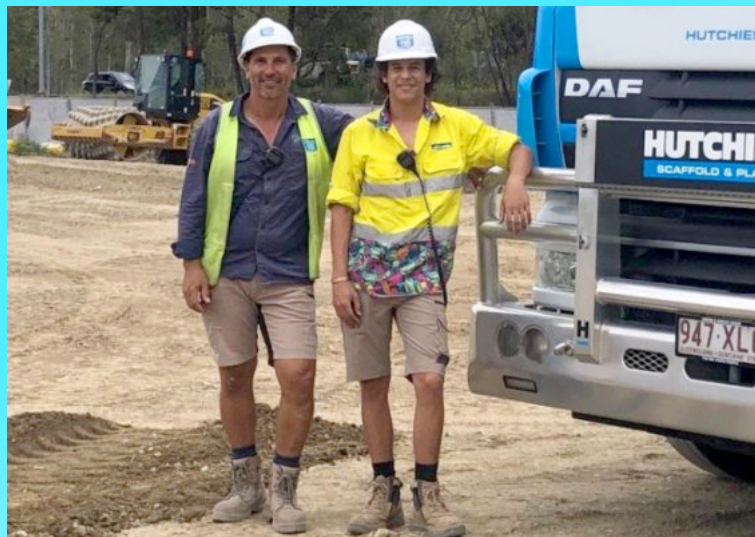
Site manager, Steve Williams, and son, Ethan, working together as team members on the Bribie Island satellite hospital site.
