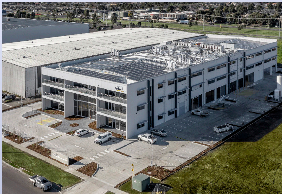
Hutchies-built Symbio Laboratories' Ravenhall facility in Victoria is now the largest testing centre in the southern hemisphere.
