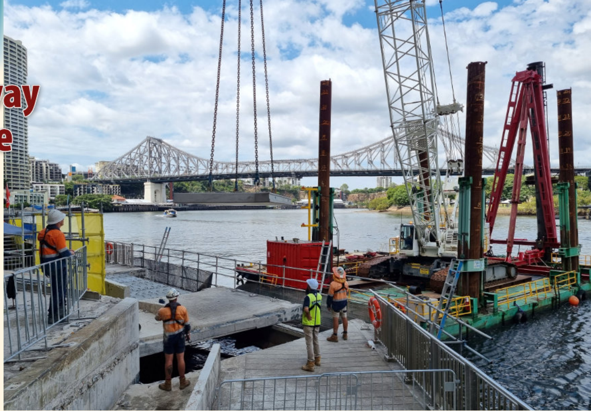
Hutchies undertaking rehabilitation work on the Brisbane City Reach Boardwalk.
