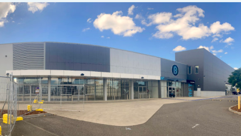
A new Kennards Self Storage facility is being created from a repurposed Masters hardware store at Roxburgh Park.
