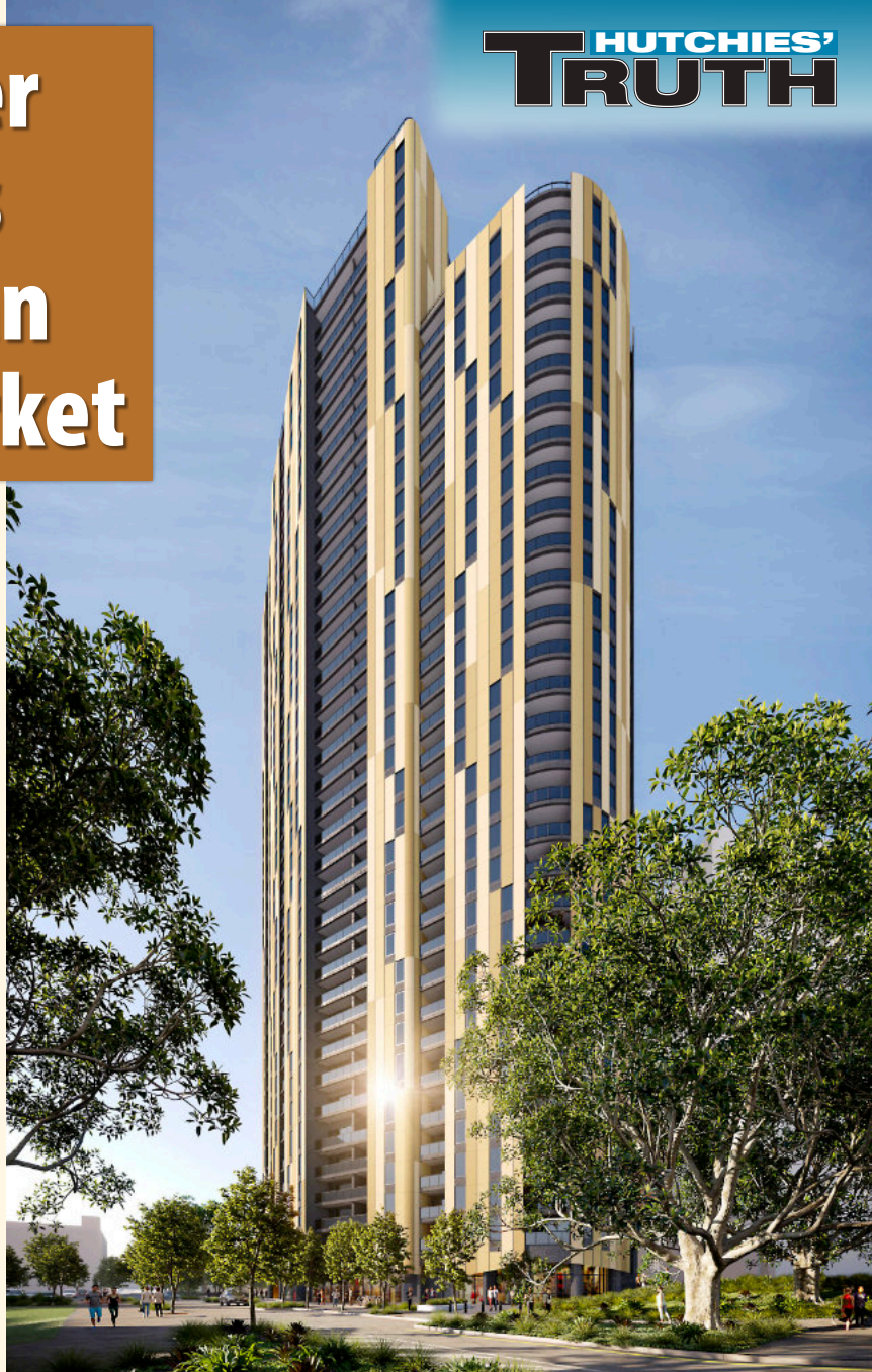
Exhibition Quarter, Lendlease's first build-to-rent project in Australia.
