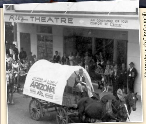
The Ritz Theatre in Ipswich ... built by Hutchies in 1939/40.
