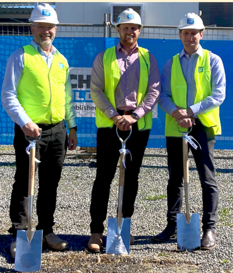
Marking the start of construction of the new silo manufacturing plant (from left) Kotzur managing director, Andrew Kotzur; Hutchies' team leader, Sean Lees; and Kotzur design engineer, Ben Kotzur.
