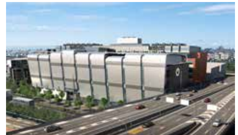
Global Switch Data Centre Ultimo, NSW
