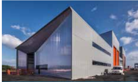
Webb Dock International Container Terminal Expansion Port of Melbourne, VIC
