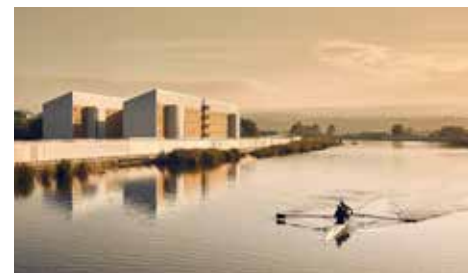
UTAS Student Accommodation Launceston, TAS
