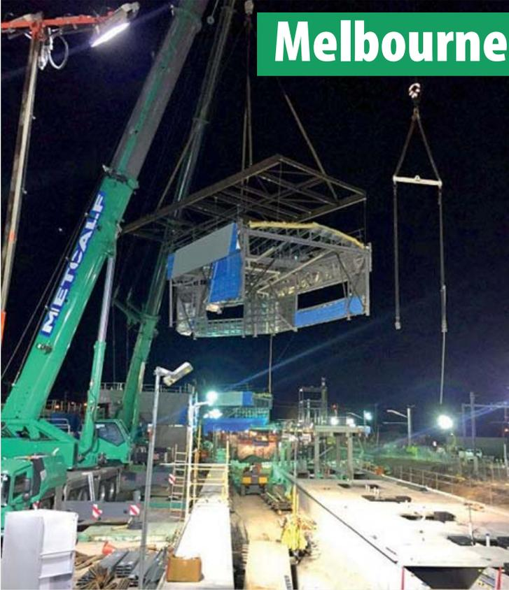
HUTCHIES has been doing some heavy lifting in Melbourne under its \$10 million contract to construct a two-storey train station, including concourse bridge and access ramp, in Bayswater, as part of a program by the Victorian Government to eliminate level crossings.
