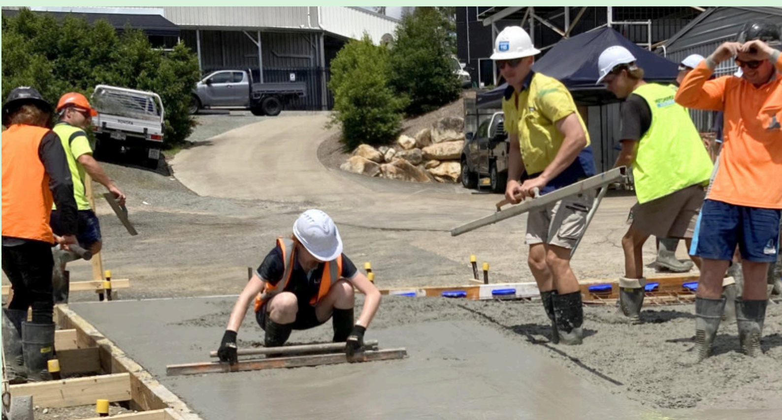
Apprentices screeding concrete under the supervision of Scott and Bryce from Creteco Queensland.
