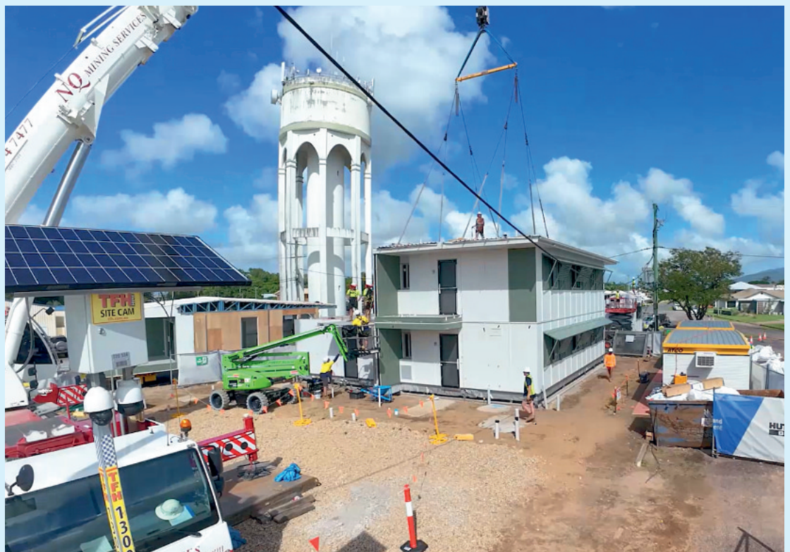
Modules from Hutchies' yard at Yatala are craned into place to create new homes for regional communities faster than conventional builds.
