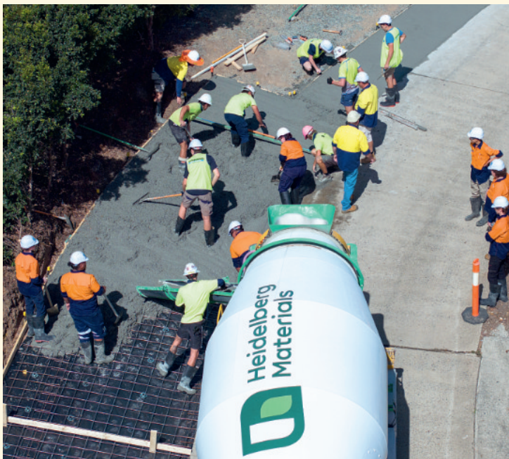
Carpark expansion underway.
