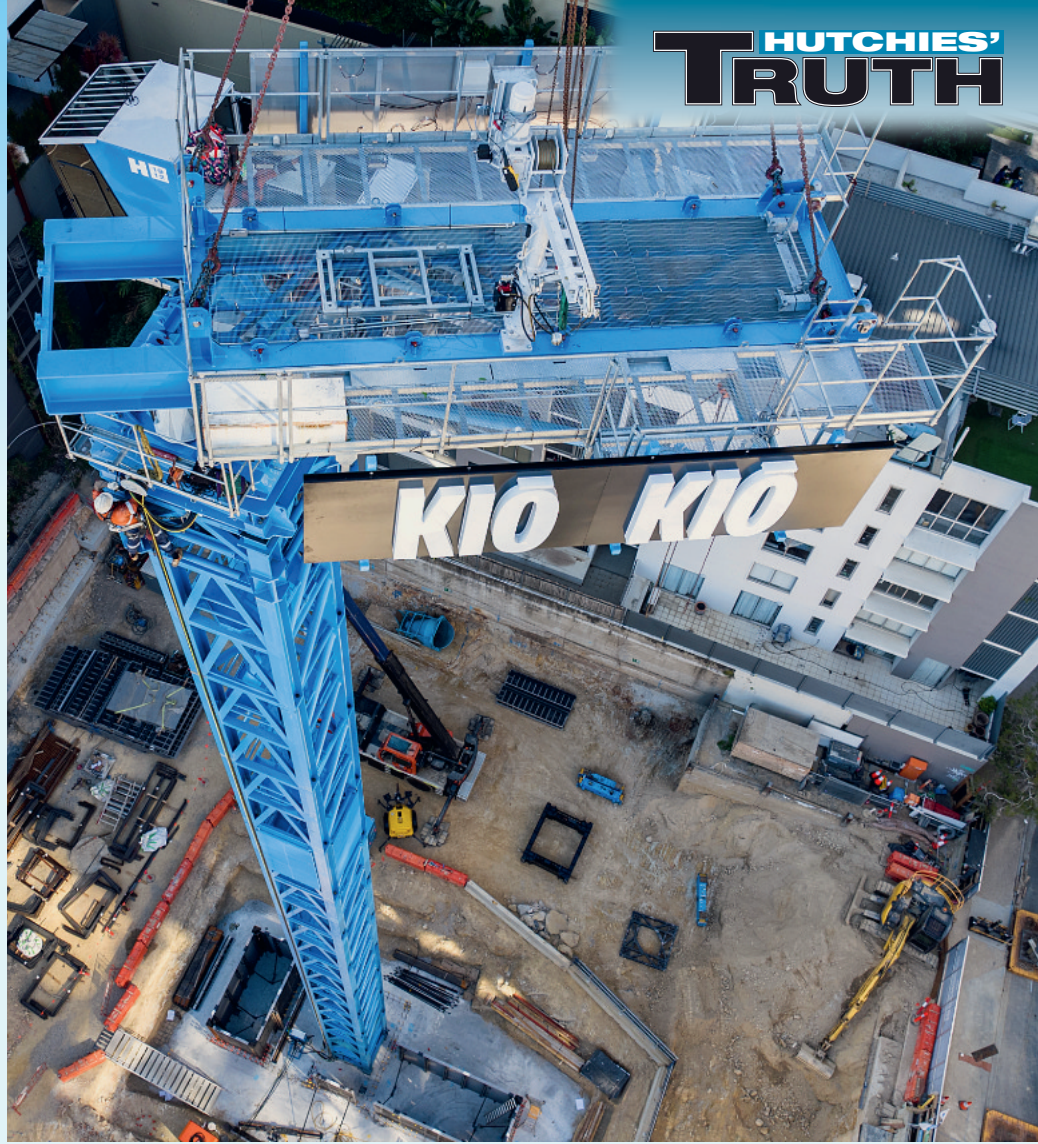
The Moritsch RTL325A-20 operating on the Halō site in South Brisbane.
