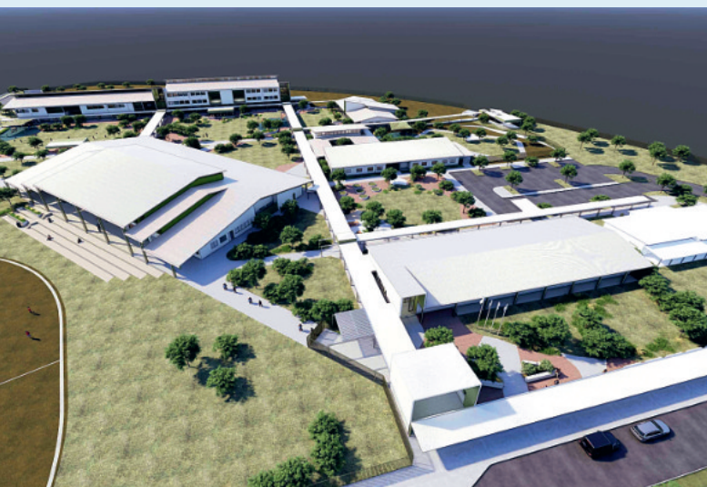
Hutchies is constructing the new Ripley Valley-White Rock State School in this growing area of Ipswich.
