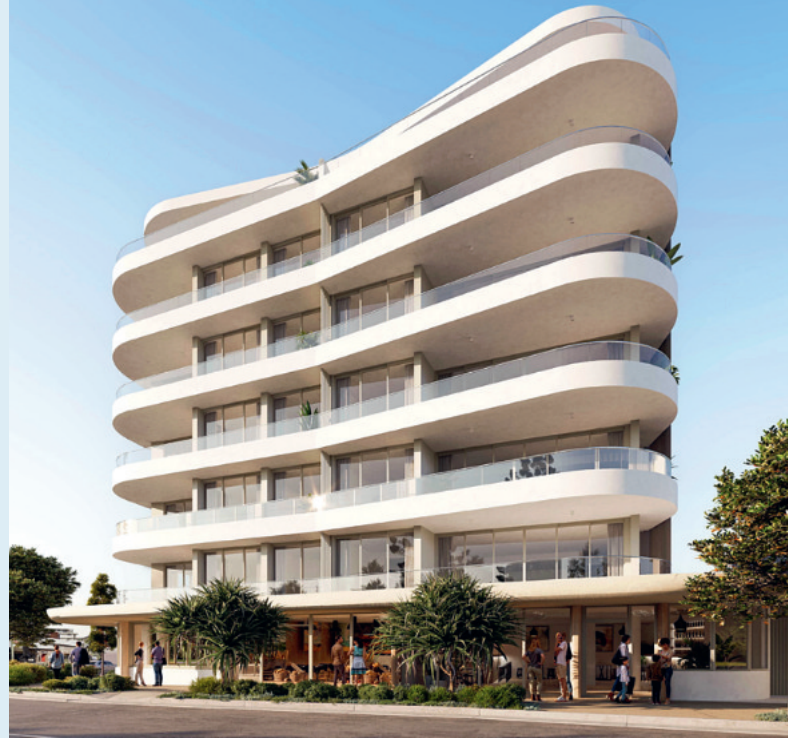
Construction is underway for Pippis, a mixed-use development within the popular beachside area of Coffs Harbour.
