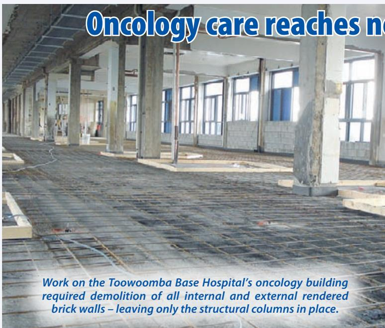
*Work on the Toowoomba Base Hospital's oncology building required demolition of all internal and external rendered brick walls – leaving only the structural columns in place.*
