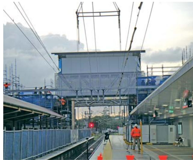
A new 11-metre footbridge was lifted faultlessly into place at the Sandgate Railway station by a 220-tonne crane.
