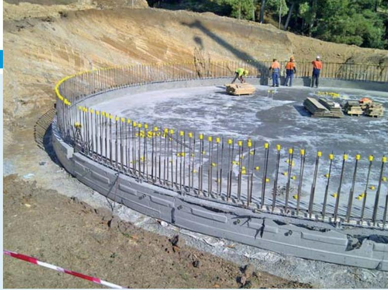
Construction is underway for a one mega-litre underground reinforced concrete reservoir at Lilydale.
