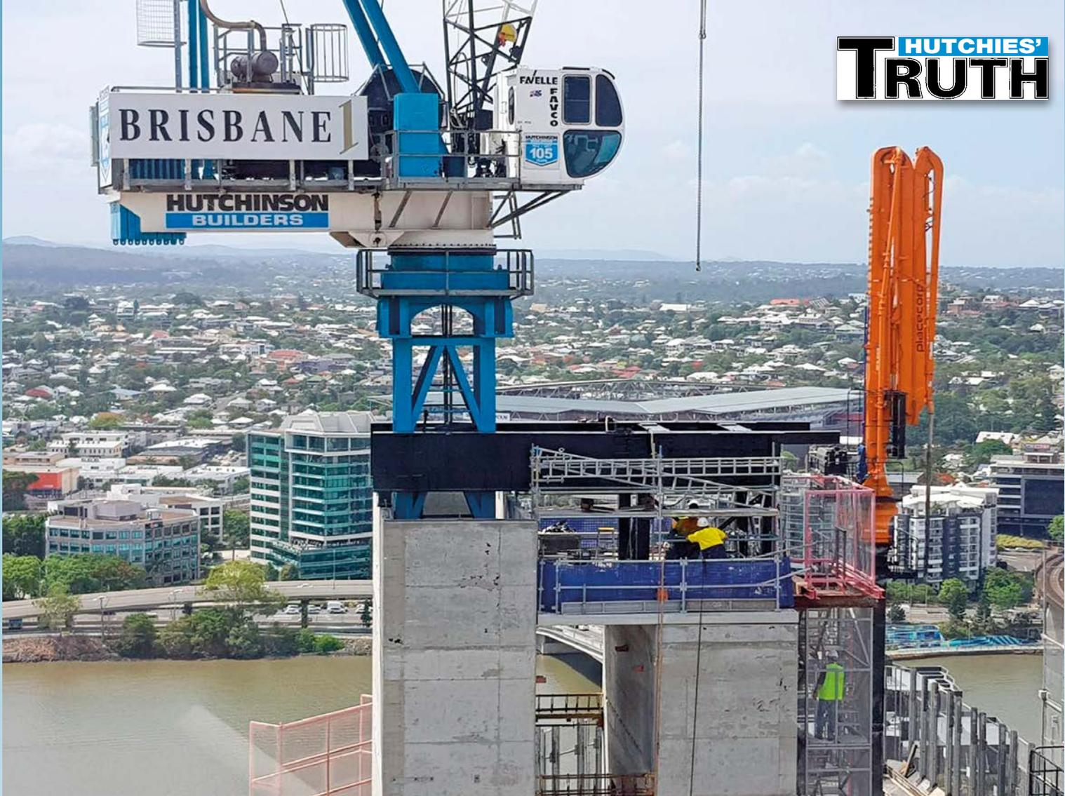
On the Brisbane One site, installation of grillage and slide beams are completed ready to accept the crane for the crane slide, freeing up access to the lift shaft.
